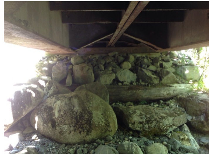
Left Bank Abutment when facing downstream
