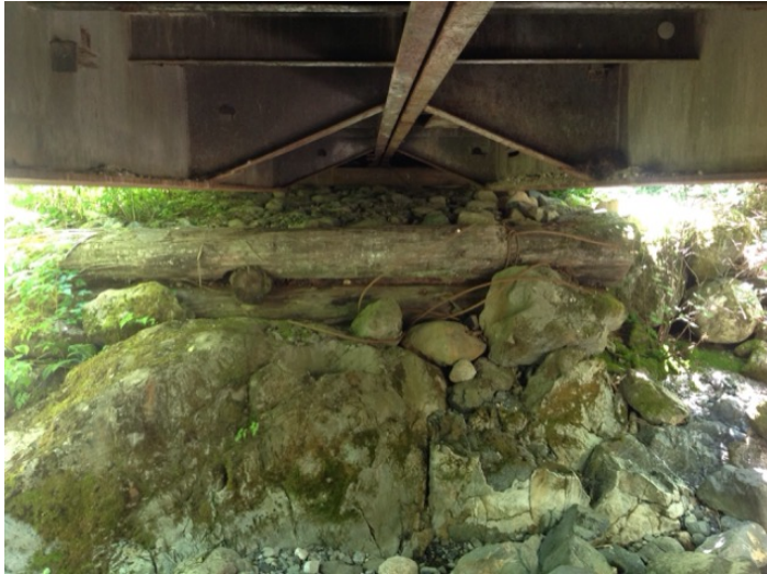
Right Bank Abutment when facing downstream
